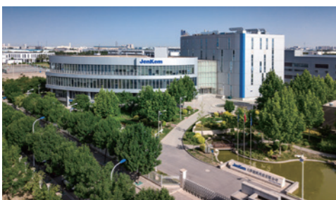
Tianjin Facility: Annual Capacity of 2MT with Batch Size up to 10kg
